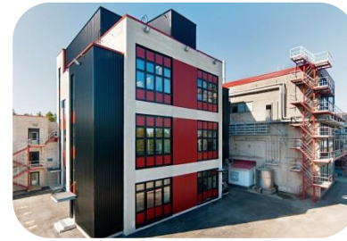
2011-2014: Expansion of Fermion's Oulu site
