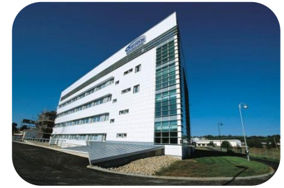
2012-2014: Expansion of Turku's pharmaceutical manufacturing plant
